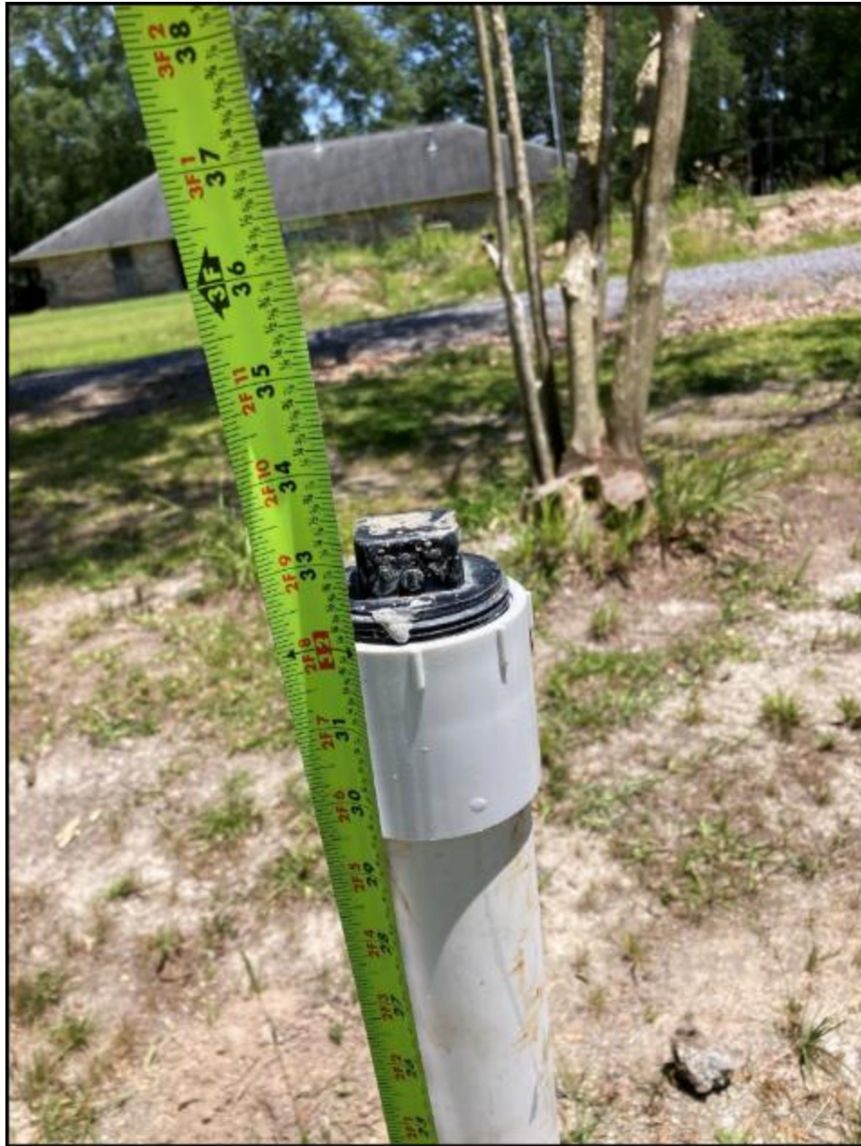
Example 1: Compliant casing height greater than 2 feet
