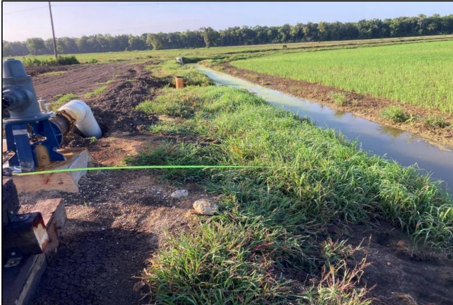
Example 21: Non-Compliant, less than 50 feet from a ditch
