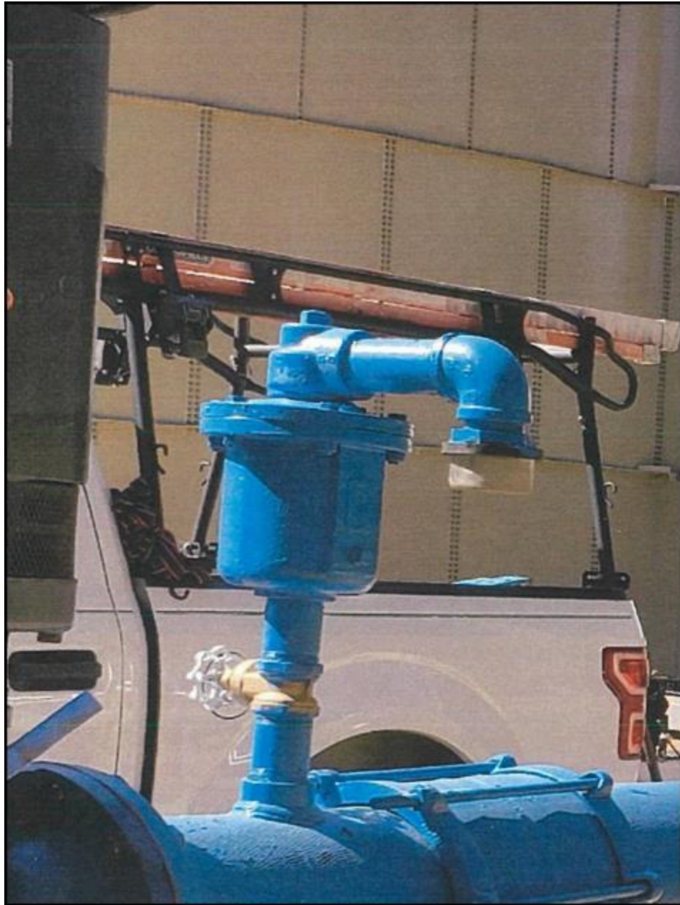
Example 11: Compliant vent is screened & turned downward
